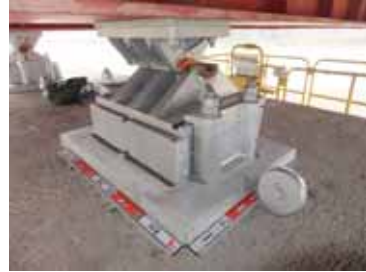
Photo 5 : Bearing failure
