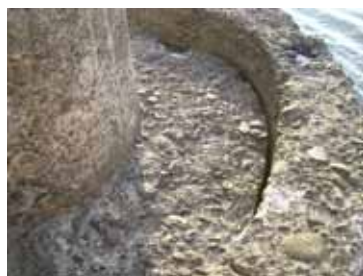
Photo 11 : Caisson damage
