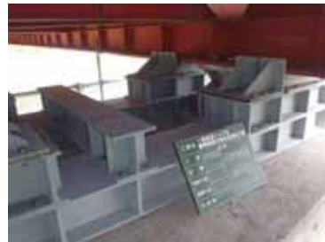
Photo 8 : Temporary repair work for bearing
