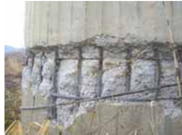
Photo 7 : Flexural failure
