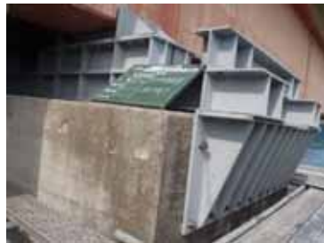
Photo 8 : Temporary repair work for bearing
