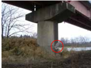
Photo 6 : Pier damage
